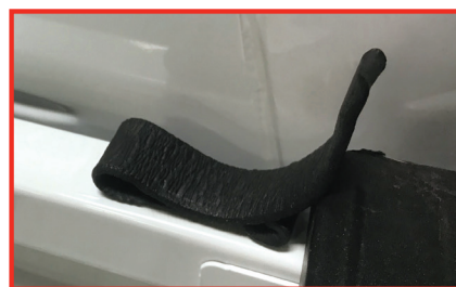
Fold putty/butyl tape into thirds, approximately 2" from bed cap.
